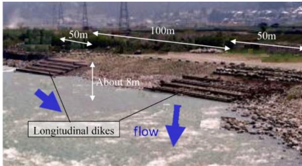
Figure 3. Longitudinal dikes for bank protection.
